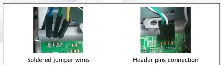
Figure 6: Physical Connections to Serial Port Headers - (Source: Author)
